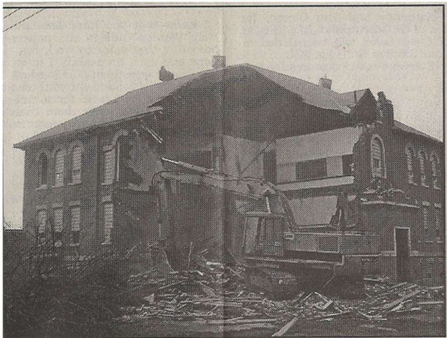
The southwest corner of the building was the first part removed.
