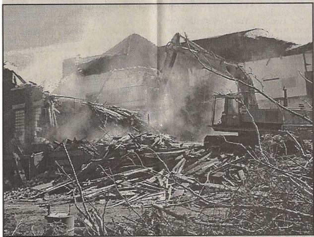
After a day of rain Thursday, work got underway again on Friday. This picture was taken from the west side of the building.
